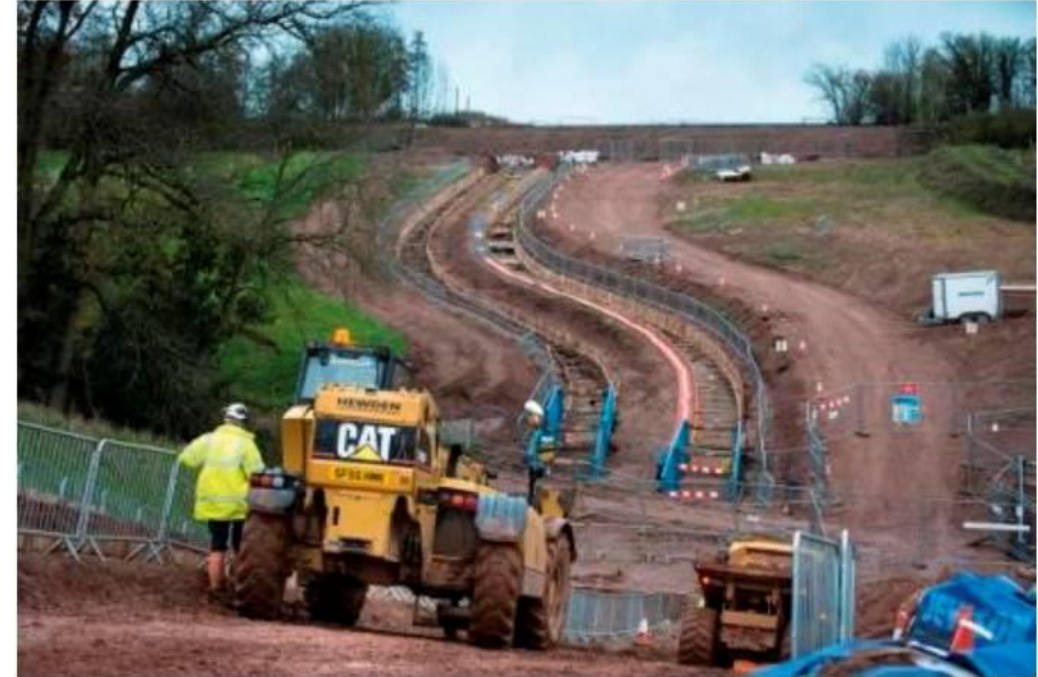
Image showing construction of two underground circuits (Parkgate requires three circuits)
